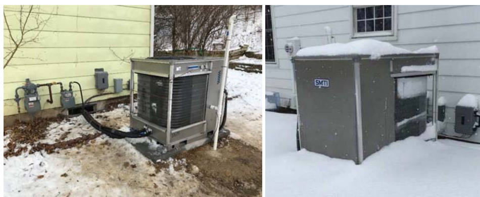
Figure 1: Pre-commercial GAHPs operating at WI demonstration sites
