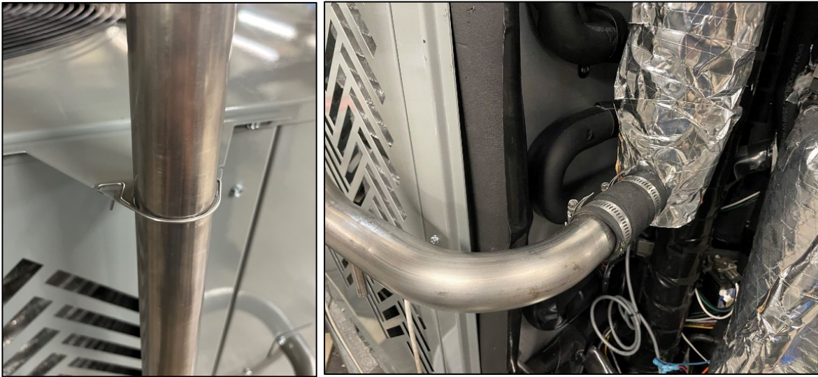
Figure 10: Flue Pipe and Bracket Installation
